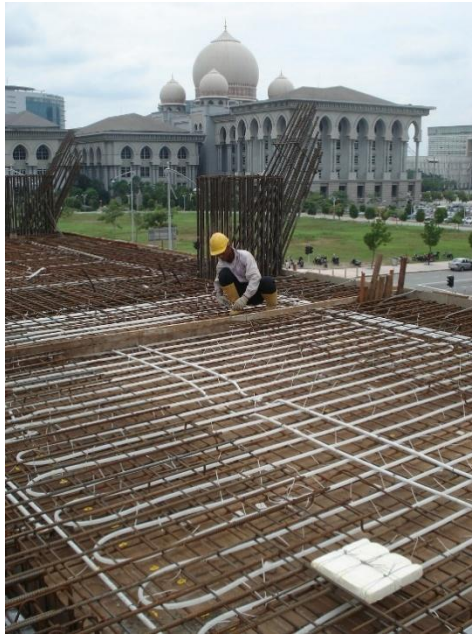
Figure 47 Radiant cooling pipes are set in the floor before concrete is poured
